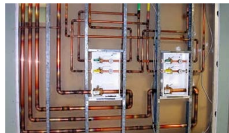
Typical commercial medical gas installation rough-in.
